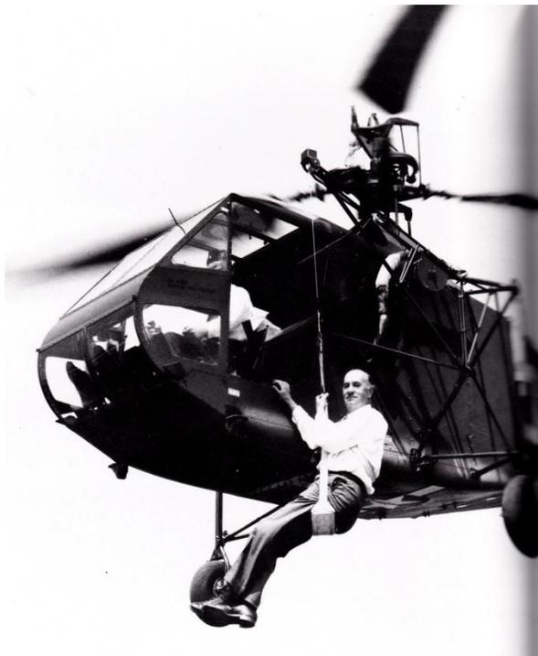
Igor Sikorsky hangs from one of the first experimental air rescue hoists during tests to develop life-saving techniques. The hoist is fitted to an HNS-1, the navy version of the R-4. One of Sikorsky's strongest beliefs was that the helicopter was destined to be a rescue vehicle. (UTC AS-346)
